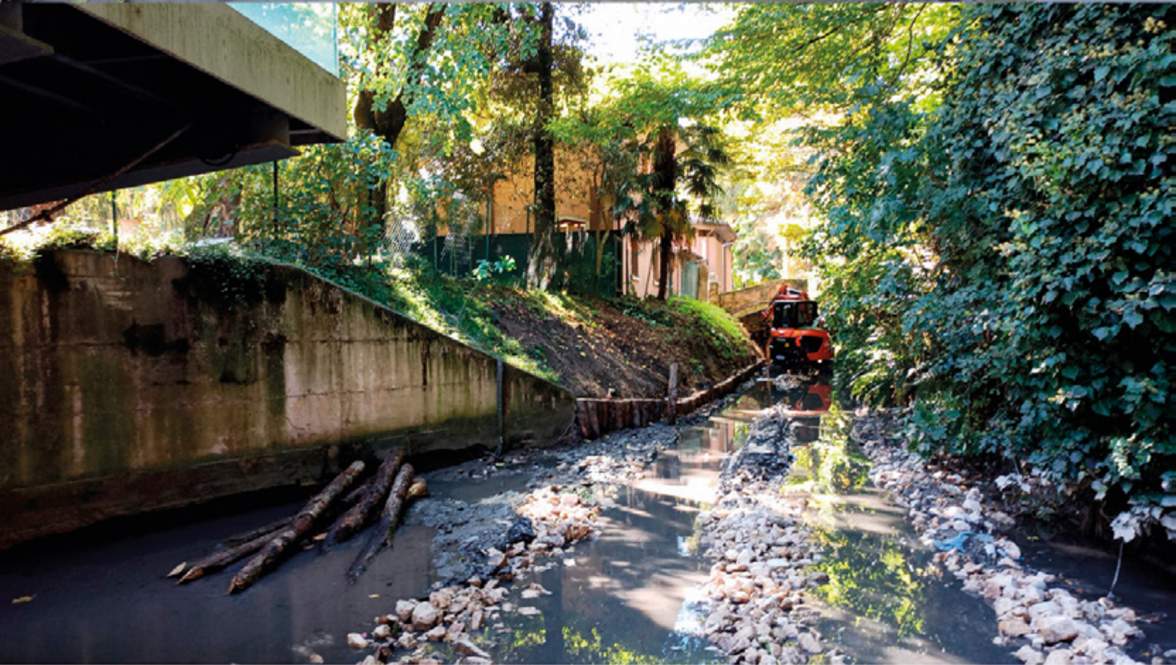
Upgrade works, dredging and strengthening of the banks of the Alicorno canal (2024)
